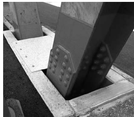
(c)補修後(あて板補修)
